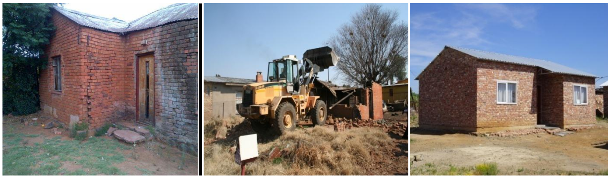
Demolition and reconstruction of better houses, MMM
